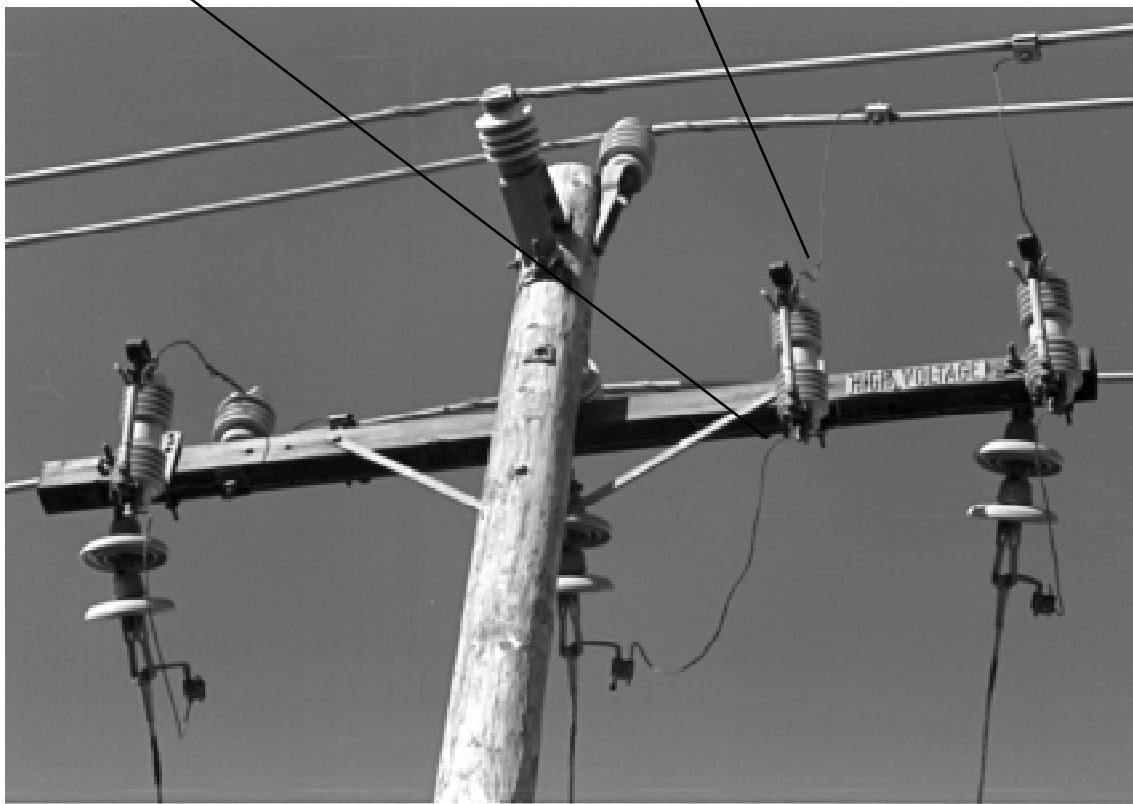
Photograph 2-1. Arm Mounted Cutout with Universal Fuse
