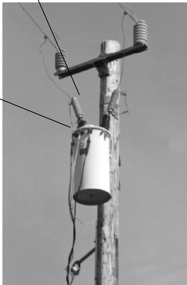
Photograph 2-3. Bushing Mounted Cutout with Open Link Fuse
