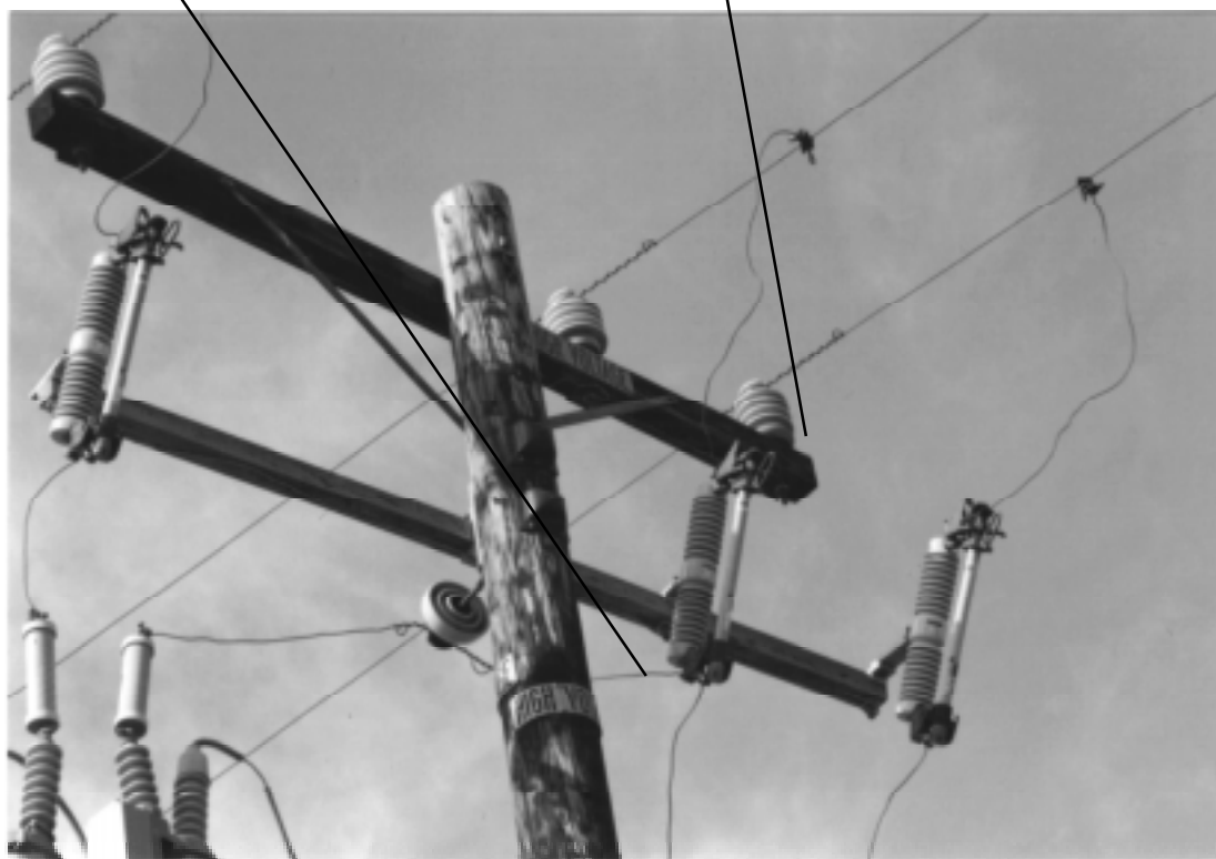
Photograph 3-5. Arm Mounted Cutout with SMU-20 Fuse
