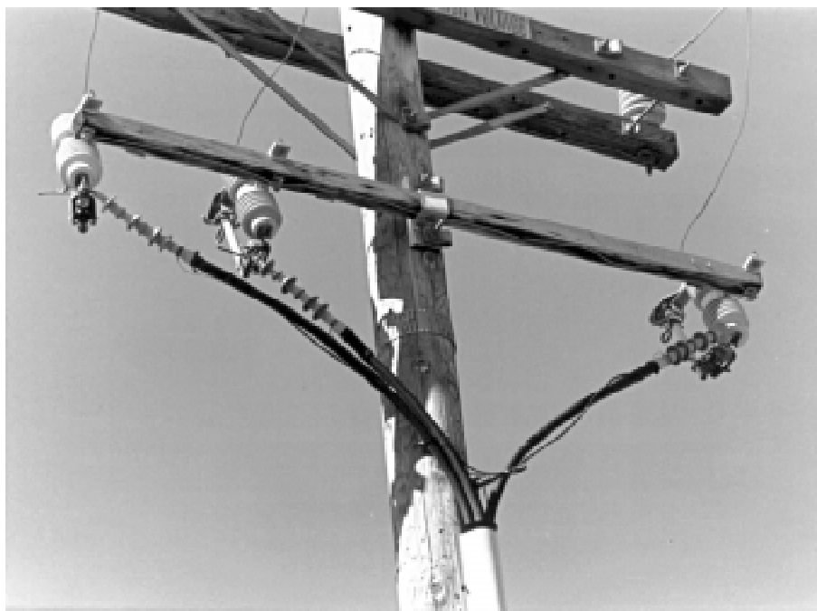
Photograph 4-6. Cable Riser with Cable Terminator
