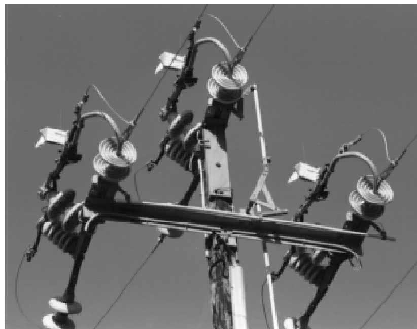
Photograph 3-9. 600 Amp KPF Air Switch Triangular Construction
