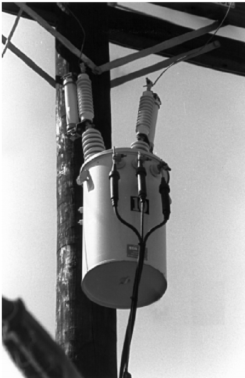
Photograph 3-15. Conventional Transformer with Exempt Fuses
