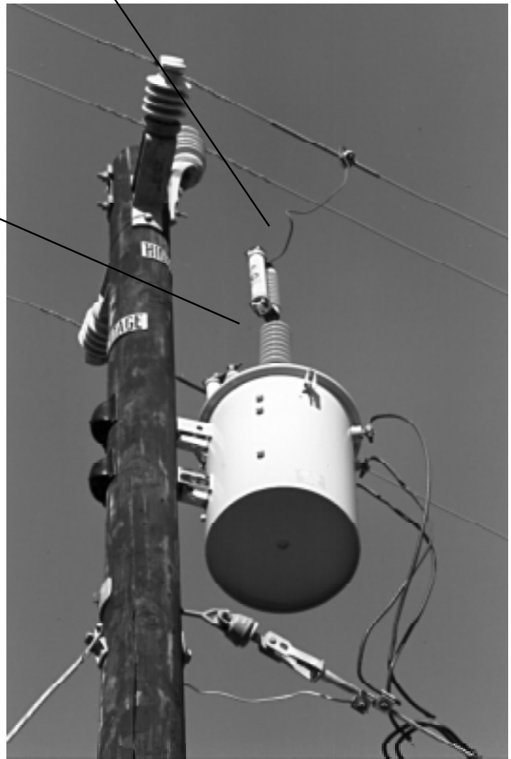
Photograph 3-3. Bushing Mounted Cutout with Non-Expulsion Fuse
