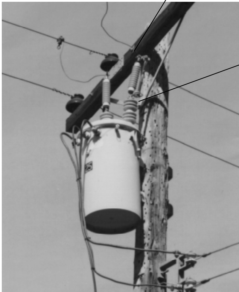
Photograph 3-4. Bushing Mounted Cutout with Liquid Filled Fuse
