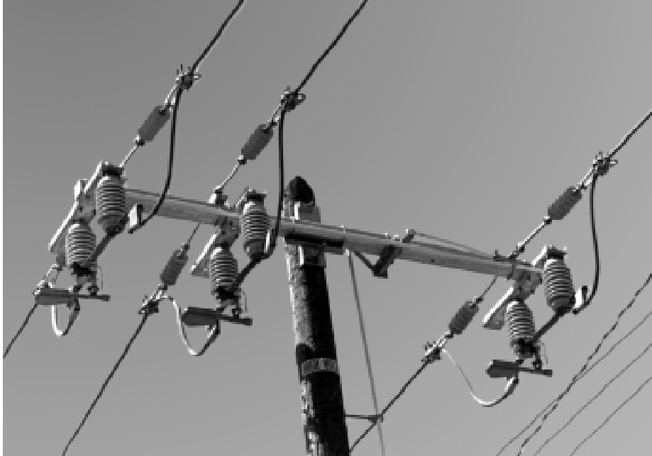
Photograph 2-17. 600 Amp Underarm Sidebreak Switch Closed Position
