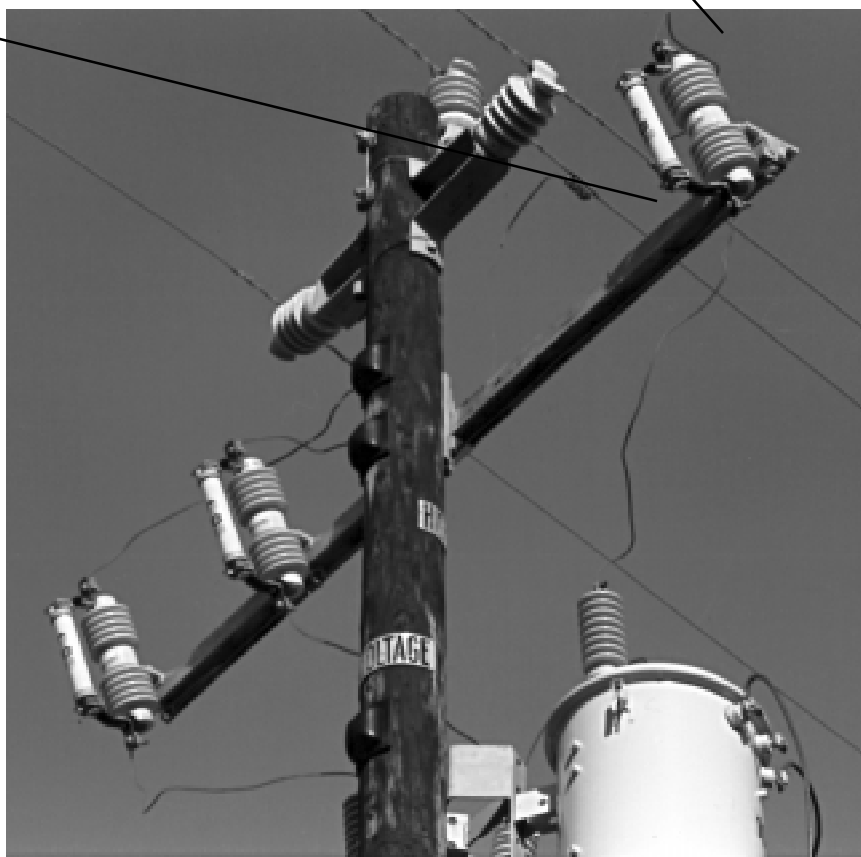
Photograph 3-1. Arm Mounted Cutout with Non-Expulsion Fuse
