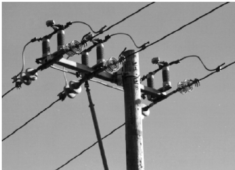
Photograph 2-19. S&C Omni-Ruptor Tangent
