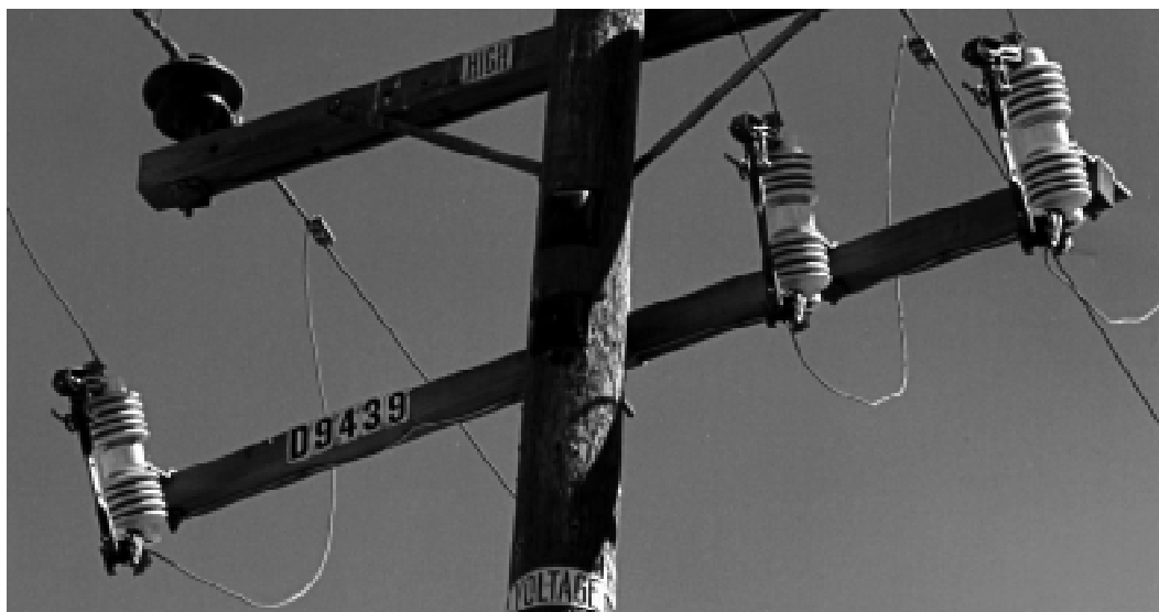
Photograph 2-5. Arm Mounted Cutout with Solid Blade Disconnect in Closed Position
