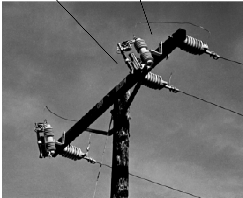
Photograph 3-7. S&C Fault Tamer Fuse
