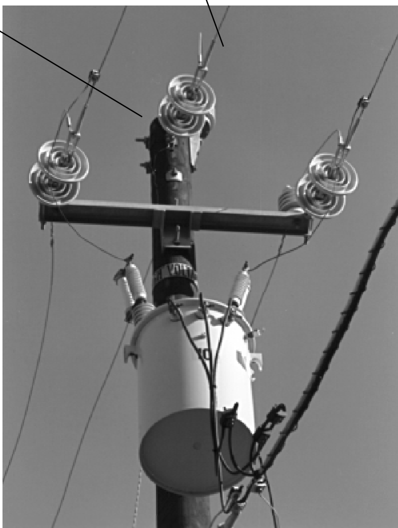
Photograph 3-26. Automatic Deadend with Suspension Insulators
