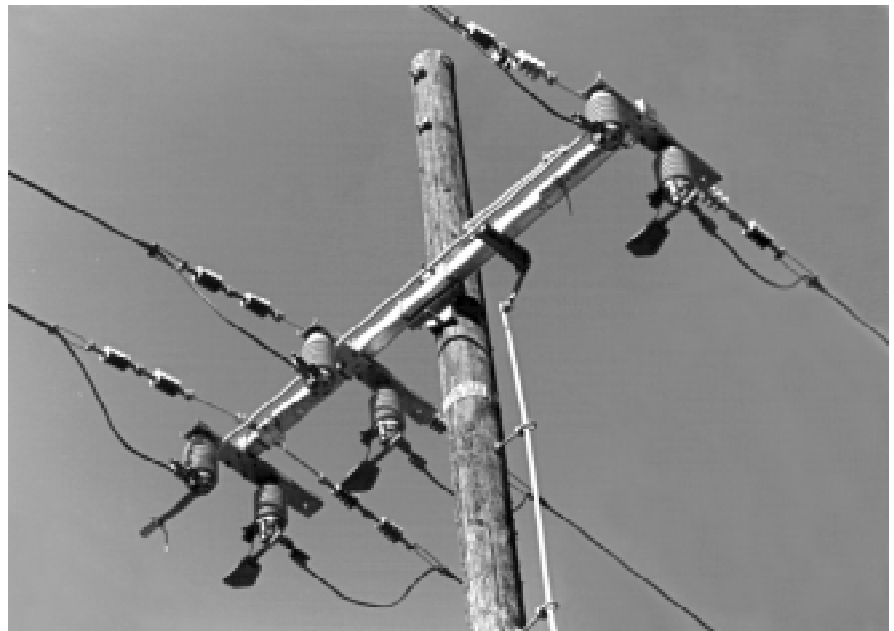
Photograph 2-18. 600 Amp Underarm Sidebreak Switch Open Position
