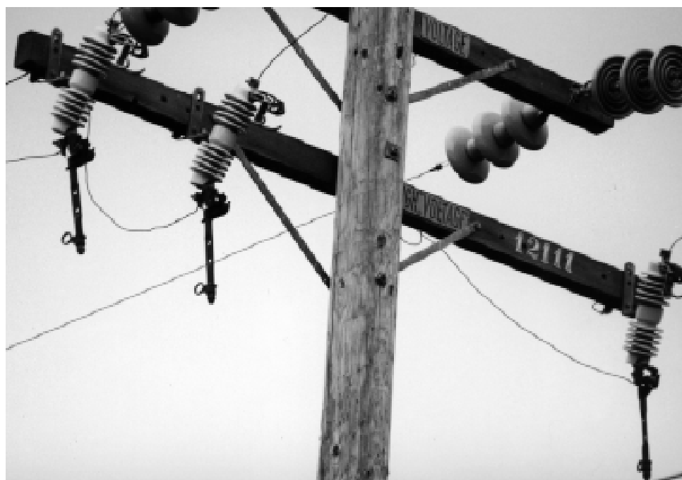
Photograph 2-6. Arm Mounted Cutout with Solid Blade Disconnect in Open Position
