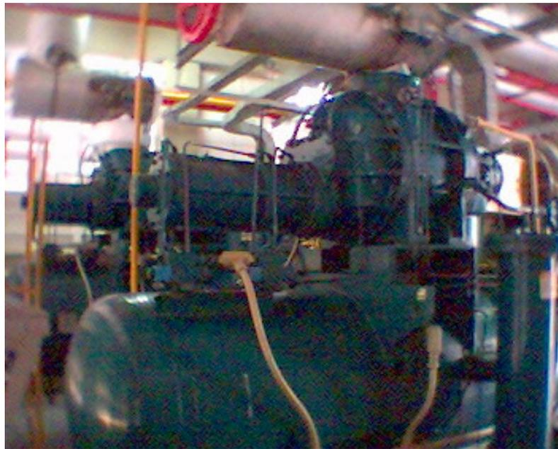
Figura 2.04 - Compressor parafuso Frick RWB-II 301,8 kW. (Mod. TDSH 233S 2334E). (-10/+35°C)
