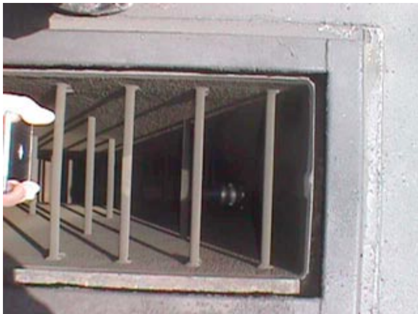
Photograph 5-16. Looking Down Exhaust Stack with Eductor Tube
