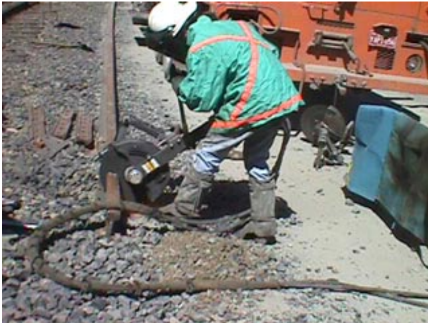
Photograph 7-17. Cutting Rail
