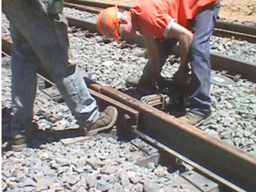
Photograph 7-12. Gas-Powered Impact Wrench in Use
