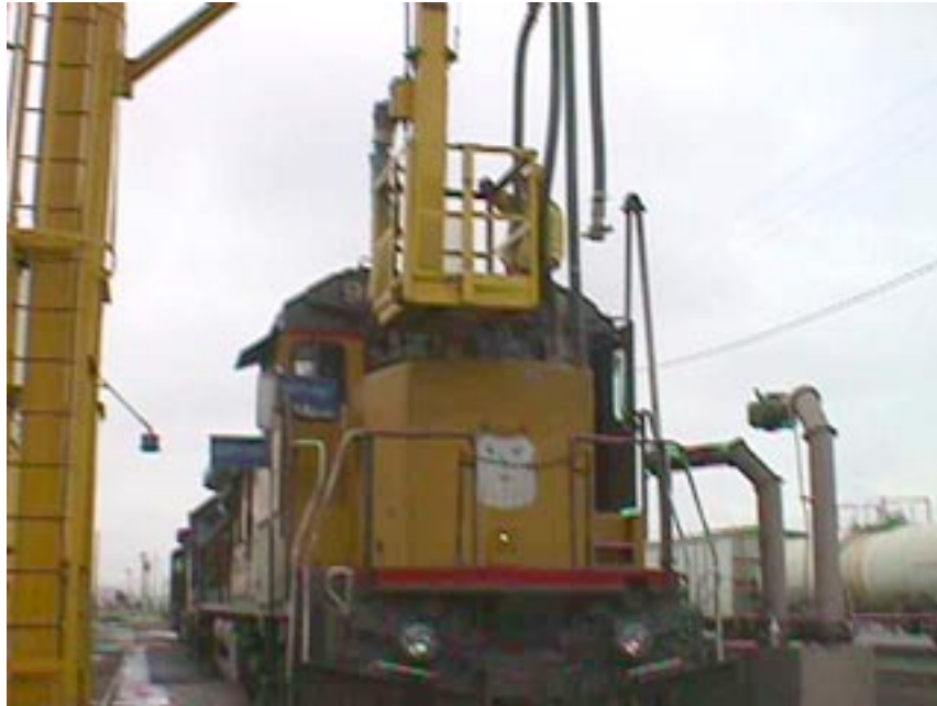
Photograph 3-5. Filling the Train with Sand
