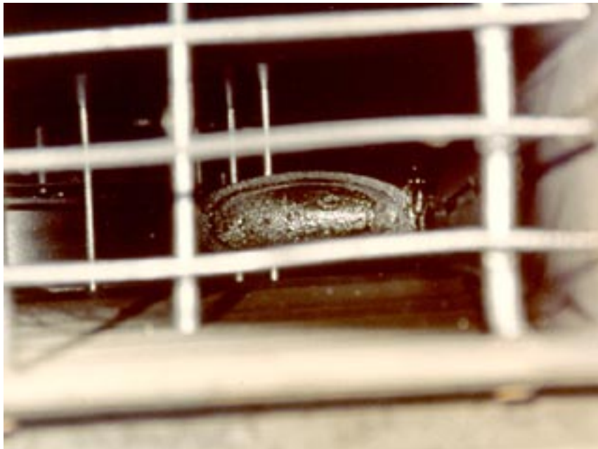
Photograph 5-14. Looking Down Exhaust Stack with Eductor Tube
