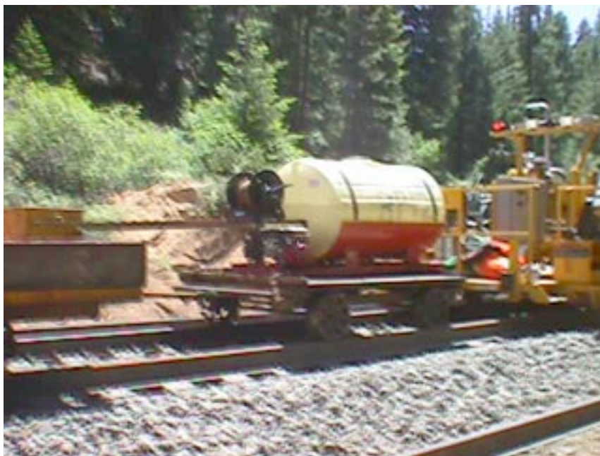
Photograph 7-14. Rail Fire Car with Working Gang
