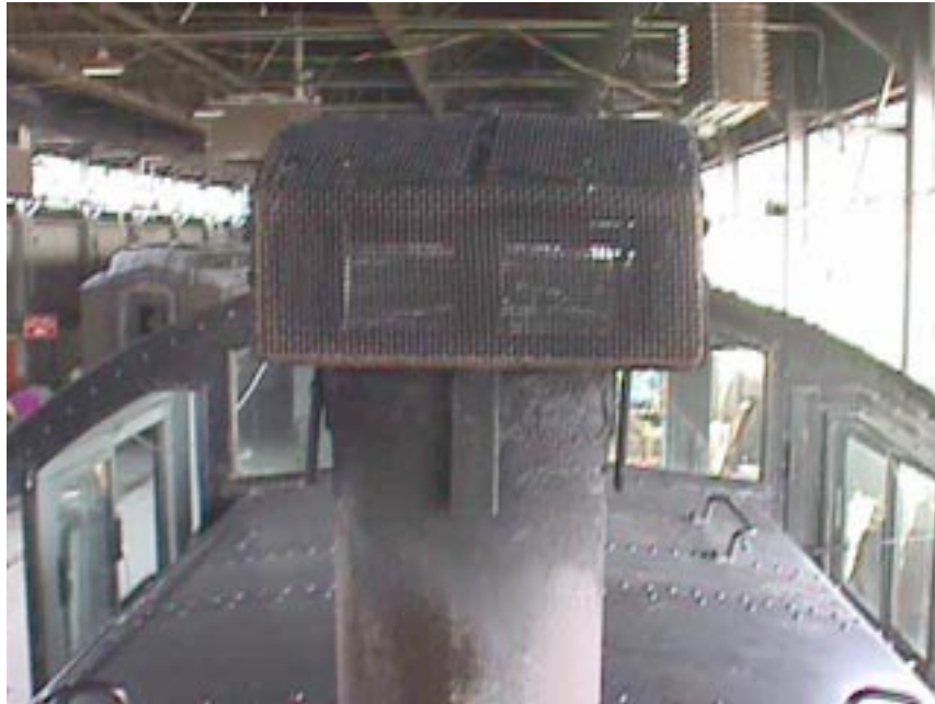
Photograph 5-5. Screen Stack (Illegal - Requires an Approved Spark Arrester)
