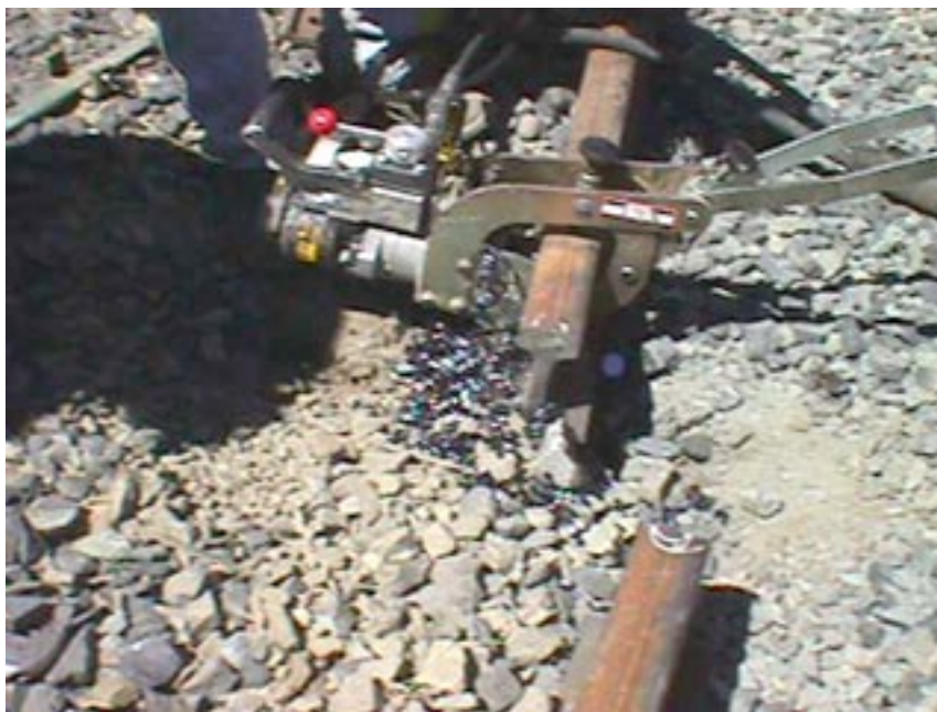
Photograph 7-19. Pneumatic Drill with Hot Shavings
