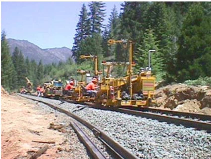
Photograph 7-4. Track Replacement Equipment Work Gang
