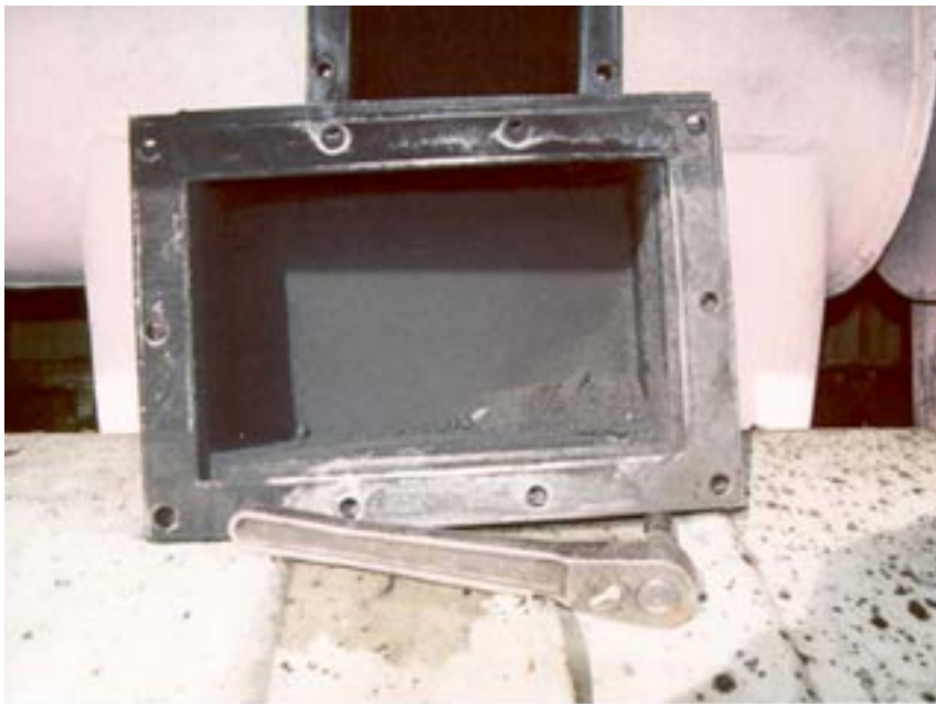
Photograph 5-7. Clean-Out Trap (Note Carbon Lower-Left Corner)
