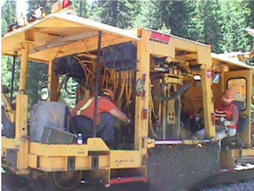
Photograph 7-3. Mechanical Spike Driver
