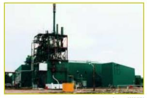
agent the higher heating value (HHV) of the fuel gas is about 6 MJ/Nm<sup>3</sup>. Enriched air, with 40% oxygen, can produce a fuel gas having a HHV of about 12 MJ/Nm<sup>3</sup> at half the gas yield. The raw gas cyclones remove 85-95% of entrained particulates.
